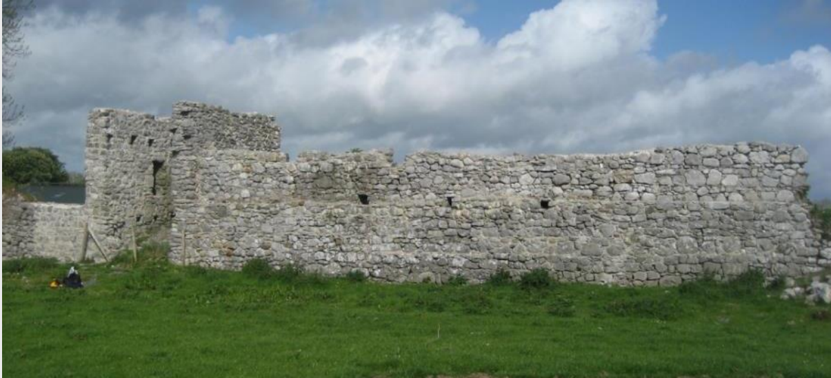
Rinn Duin - Tower 3 on Completion
