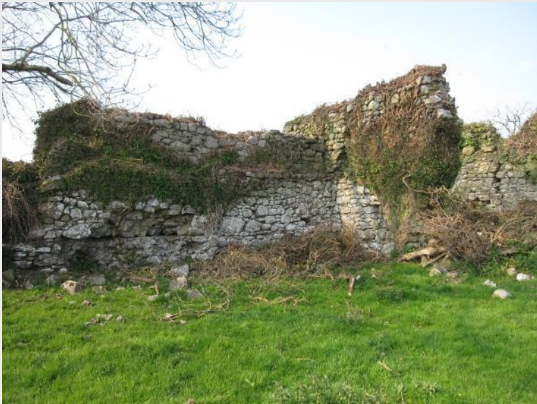
Rinn Duin - Gatehouse Pre-Works
